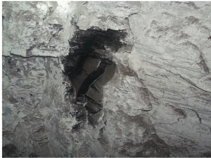
Fig 6.7: Dolomite painted coal wall
